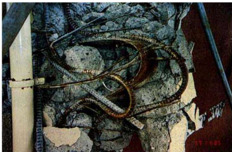
(a) 柱のせん断破壊
