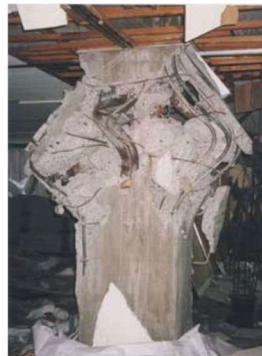
(a) 柱のせん断破壊
